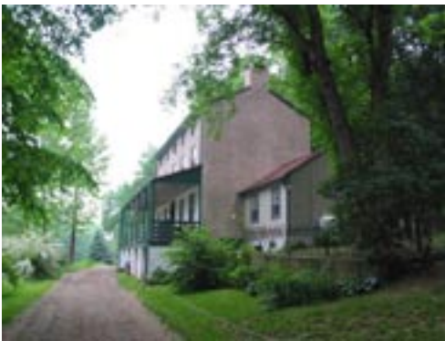
Locktender's House at Lock 60, Mont Clare
