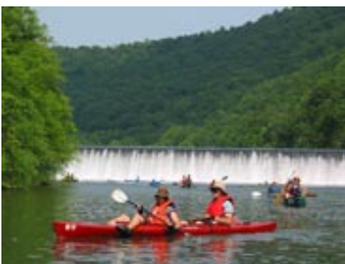
Kernsville Dam, Hamburg
