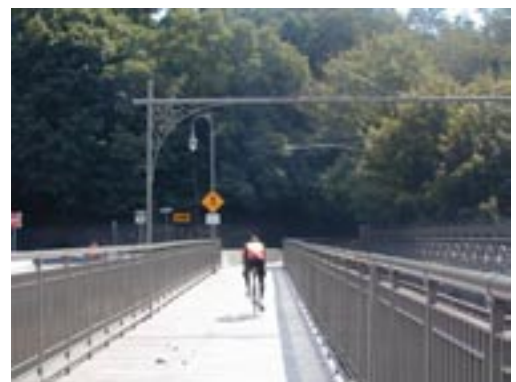
Strawberry Mansion Bridge, Philadelphia
