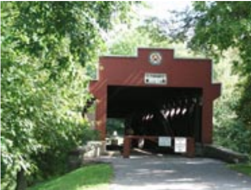
Red Bridge over the Tulpehocken Creek, Bern Township
