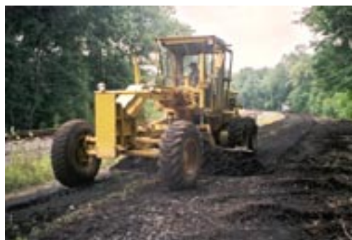
Thun Trail Construction
