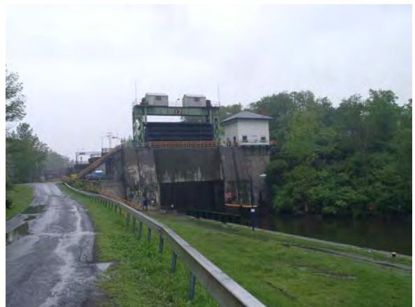
Canalway Trail at Lift Lock
