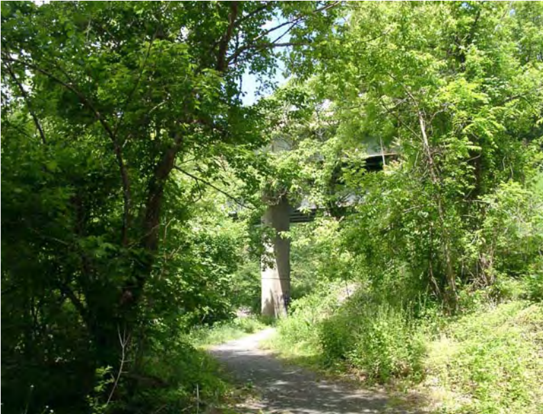
Existing Path under Highway bridge
