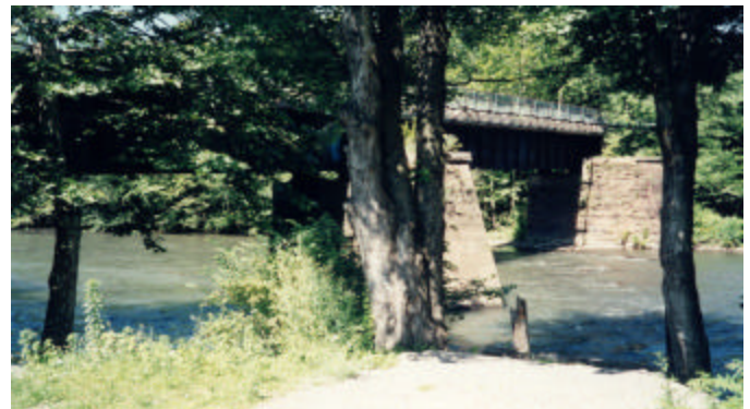
Figure 1.1 The Hamburg/Tilden pedestrian bridge.
