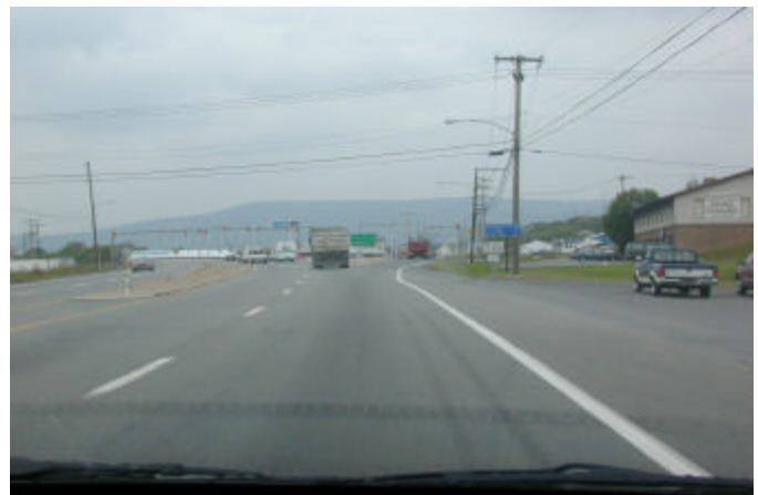
Figure 1.6 The intersection of Route 61 and Fourth Street looking north on Route 61.
