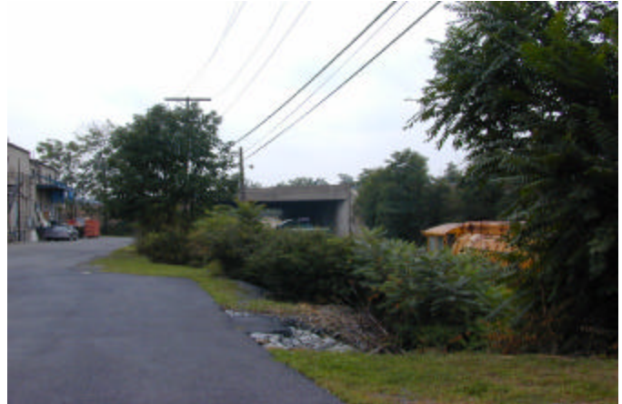
Figure 1.2 The Blue Mountain Rail Road underpass in southern Hamburg.
