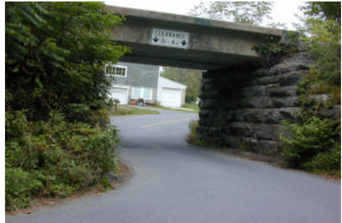
Figure 1.8 The narrow railroad underpass on Five Locks Road
