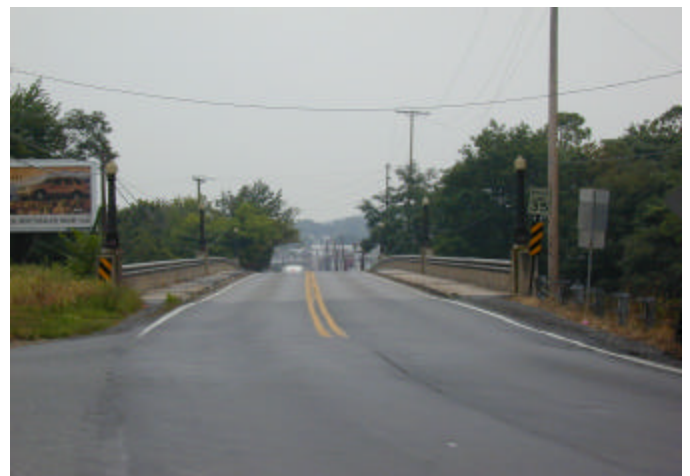
Figure 2.2 The State Street Bridge looking east toward Hamburg.
