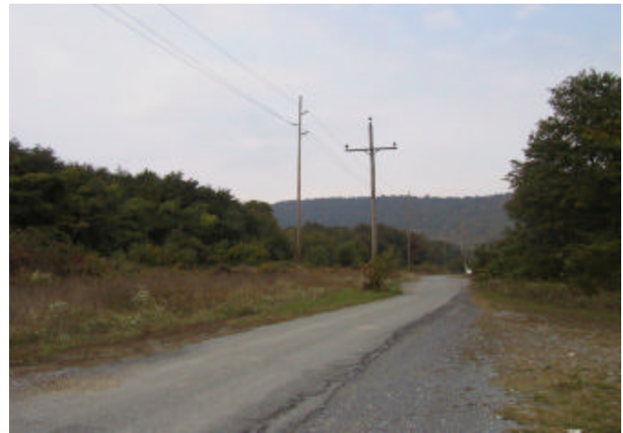
Figure 3.2 A view of the dam facility access road, just below the dam.
