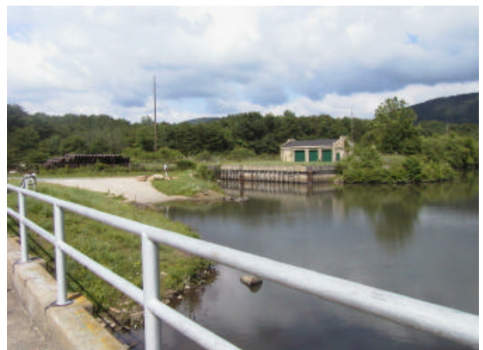
Figure 3.9 This is a view of the BAMR boat launch and maintenance facilities from the Kernsville Dam.
