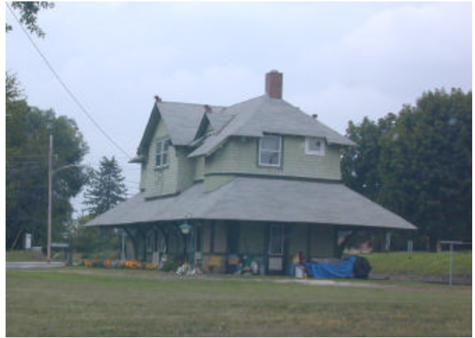
Figure 4.7 The original railroad station in Shoemakersville continues to be occupied.
