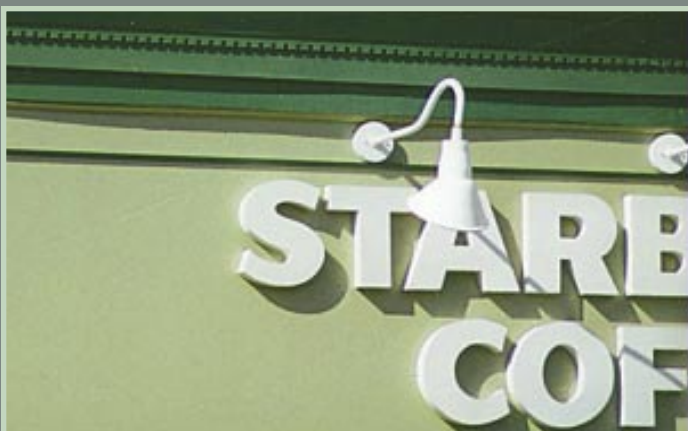
Large simple mounted letters, with exterior light fixtures, cast strong shadows and are easily read.
