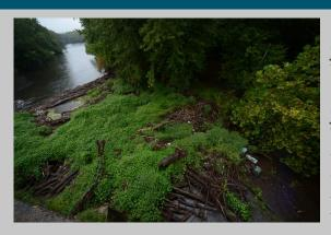
Contractors have begun removing a log jam from under the Douglassville bike/pedestrian Bridge along the Thun Section of the Schuylkill River Trail, just west of Morlatton Village. The build up of logs, debris and trash along the bridge piers has created a hazard for paddlers in the river, and, if allowed to continue, could undermine the bridge.
