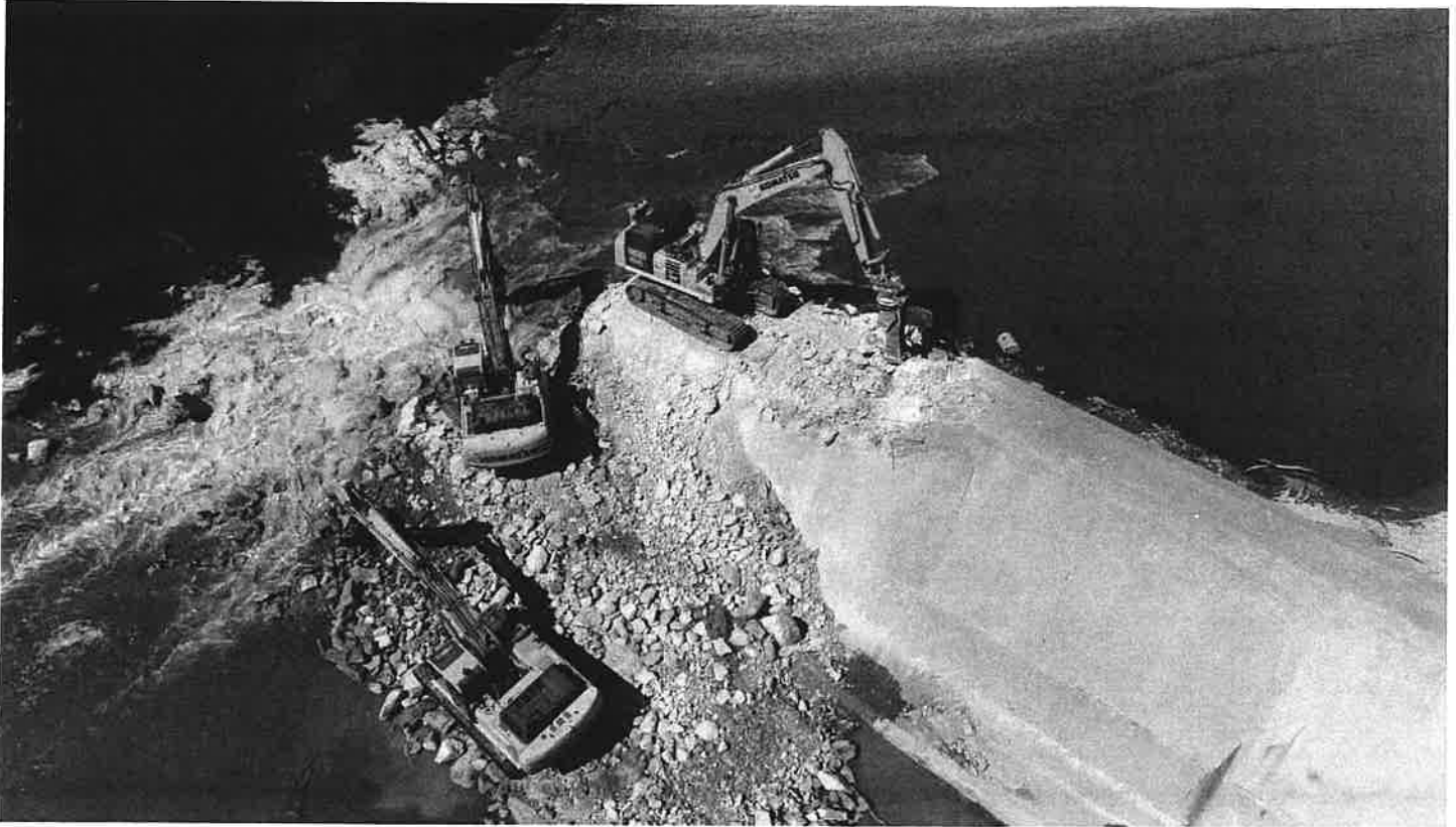
Removal of Spillway (Ballville Dam, Fremont, OH)
