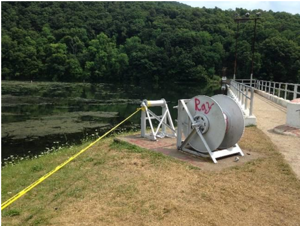
3. Dredge pipe and launch capstan
